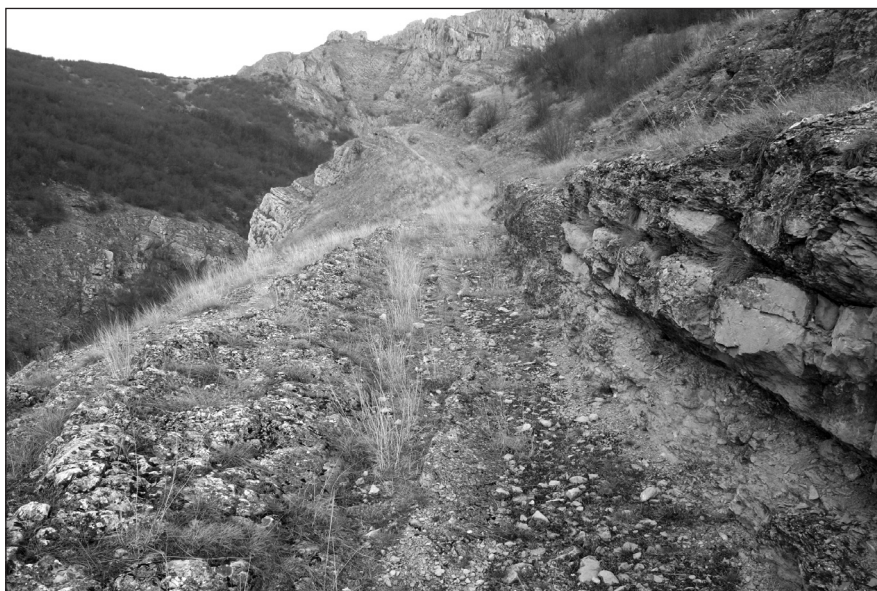
Fig. 1 Remains of the road with visible embankments at the entrance to the Svrnjiški Timok gorge
